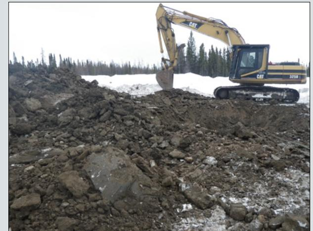
A-002-D/094-P-13 (WA# 21051) was abandoned in December 2013 and cut and capped in February 2014. (Top to bottom) Workers plug the well; the well is capped, and the area around the well is re-filled with soil.
