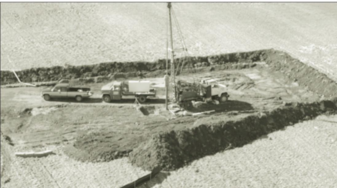
*A dirt berm is constructed as a preventive measure in the unlikely event of an uncontrolled release. This is a standard procedure of oil and gas drilling operations throughout the province, and was used as part of CBM exploration. Photo by Boomer Jerritt, courtesy of Priority Ventures Ltd.*
