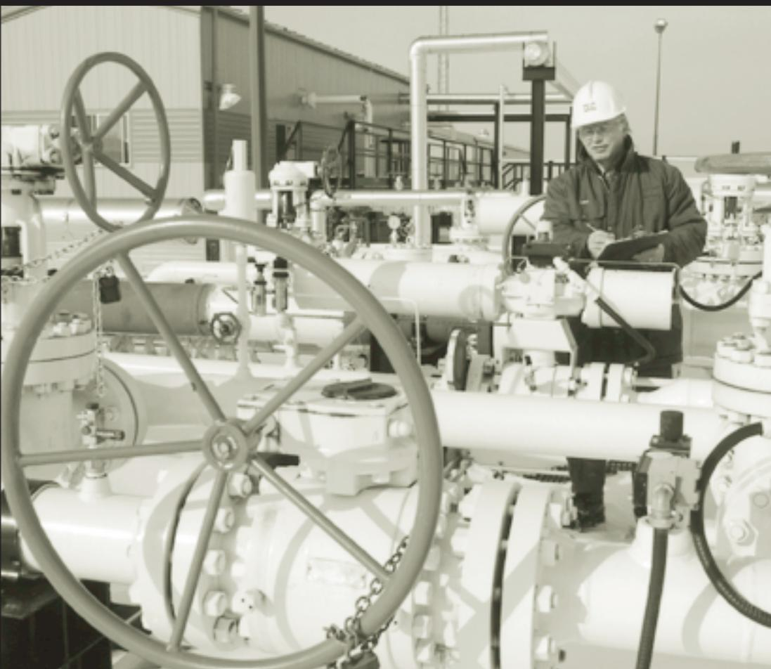
*OGC inspectors are required to regularly inspect oil and gas facilities. Pictured here is Operation Inspector, Len Barteaux. Mr. Barteaux is conducting a routine inspection of the Emergency Shutdown Devices (ESD) at the Williams Energy Taylor Pump Station. ESD equipment will activate in the event of pressure changes.*
