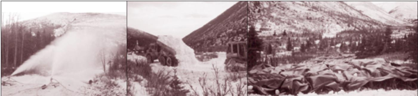
*Murphy Oil Company Ltd. used machine-made snow for stream crossings and access roads. This allowed access to sites in low snow conditions with minimal disturbance.*
