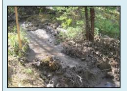
Horizontal boring release of drilling mud to surface, approximately 10M<sup>3</sup>; within ROW
