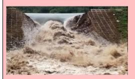
Massive dam slope failure or dam breach or dam overtopping or piping (internal erosion) is occurring and progressing at high pace where control or stoppage is impossible.
